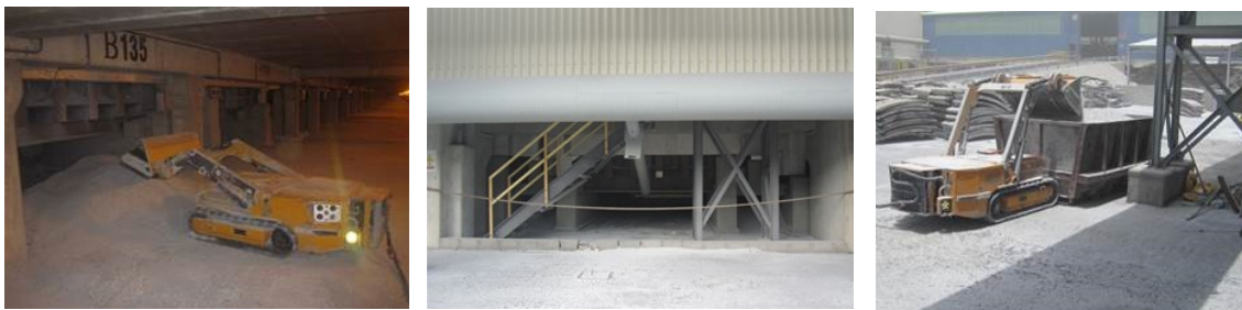
Figure 3. Before and after - basement with excess material (left), clean basement (middle) and handling equipment (right).
